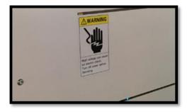
**Danger:** Potential immediate danger High voltage can cause an electric shock Turn off before servicing
